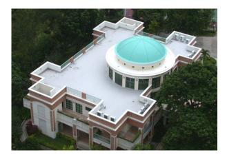
TamSeal 23E is a single-component polyurethane membrane used for long-lasting waterproofing. TamSeal 23E is a liquid-applied, highly elastic, cold applied and cold curing. It cures by reaction with ground and air moisture. Its enhanced UV resistant properties enable this product to be used as a weatherproof membrane while remaining flexible and durable, offering long-term protection to substrates against climate conditions. It is suitable for use over horizontal and vertical surfaces.
